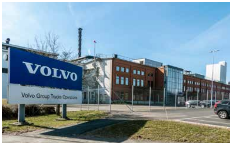
The investment in the foundry in Skövde will lead to greater flexibility regarding products and materials.
